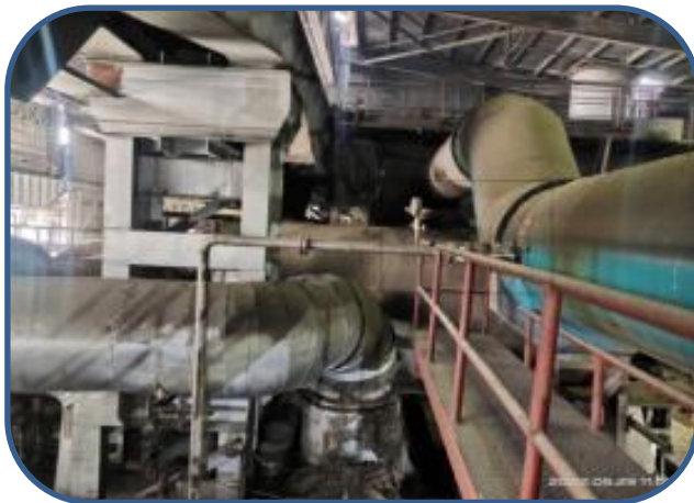
Oxy Enrichment Line Joint with Combustion Air Line
