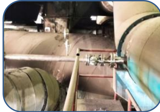
Oxy Enrichment Line Joint with Combustion Air Line
